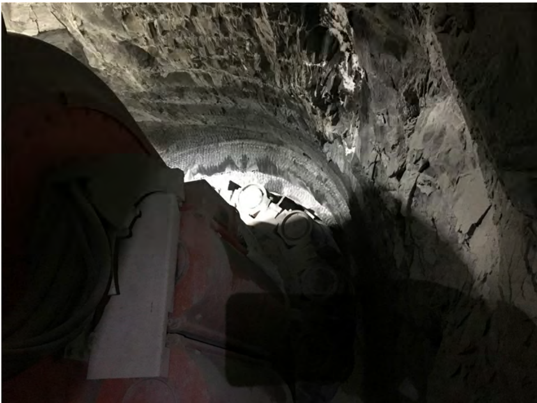
MX650 Rapid Mine Development System (RMDS) in operation.
